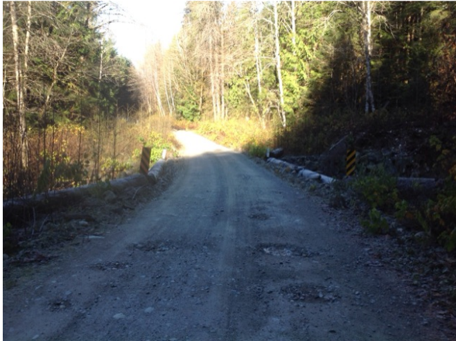
Approach from Left Bank when facing downstream
