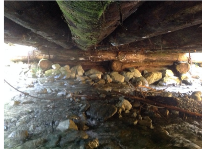
Left Bank Abutment when facing downstream
