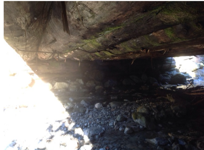
Right Bank Abutment when facing downstream
